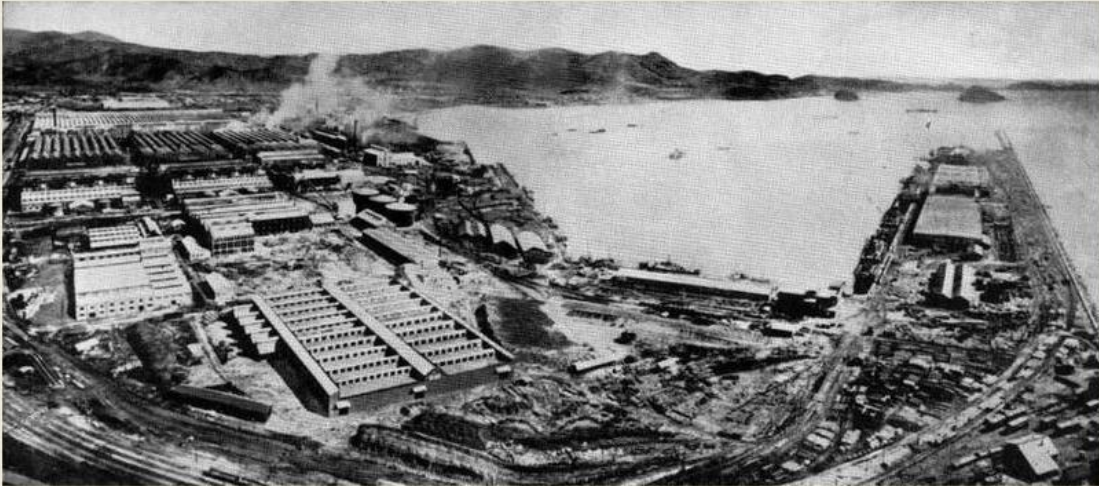
Heungnam, North Korea: modern industrial city built by Japan
