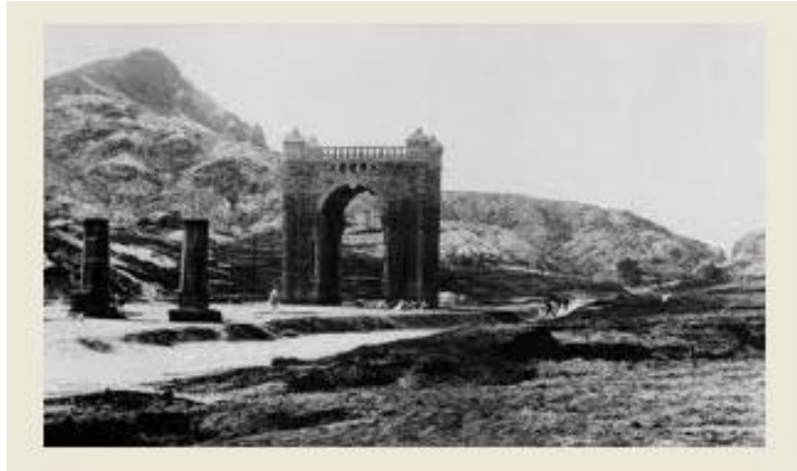
Dongnim (Independence) Gate: Pillars from the former gate (Yeongeun Gate), a symbol of subservience, remain
